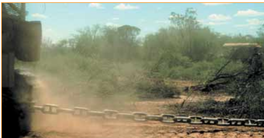
▲ Two dozers are required to pull the chain.
