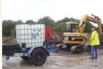
Wash down, on site if possible
